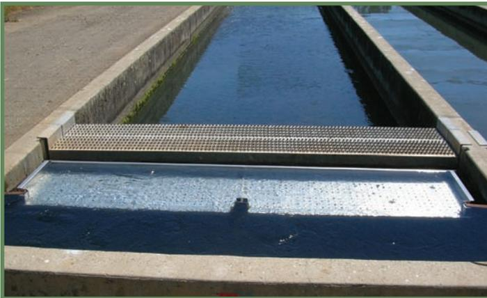
The Low Head Oxygenator (LHO) System super-saturates water with oxygen without using high pressure pumps or compressed oxygen typical of other oxygenation equipment. PR Aqua customizes LHOs to meet desired oxygenation results, footprint restrictions, and flow rate requirements.
