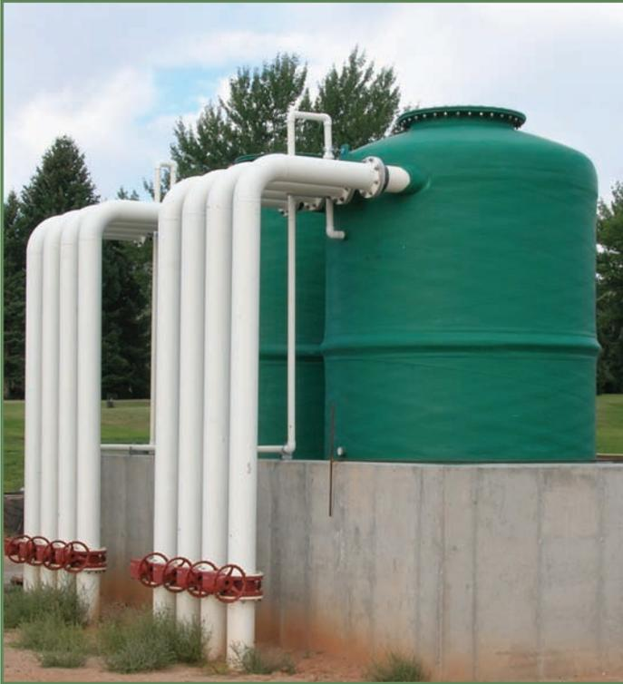
The PR Aqua Vacuum Degasser is an open bottom column designed to be installed in a header tank containing water to a required depth. Water enters the vessel through a sealed top and cascades down into the vessel. A vacuum pump or blower creates lower pressure within the vessel thereby releasing gases from the water into the atmosphere. Stripped water is discharged into a header tank and is ready for further treatment if required.
