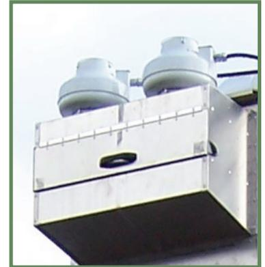
Water enters the vessel from the top orifice plate and cascades down through a Carbon Dioxide Stripper. Blowers, sized specifically for desired flow rates and carbon dioxide removal, force fresh air across water droplets. This process drives off carbon dioxide and absorbs oxygen until the dissolved gases are close to saturation. Treated water flows into a stilling chamber and is delivered to the top of the LHO chamber where water is supersaturated with oxygen.
